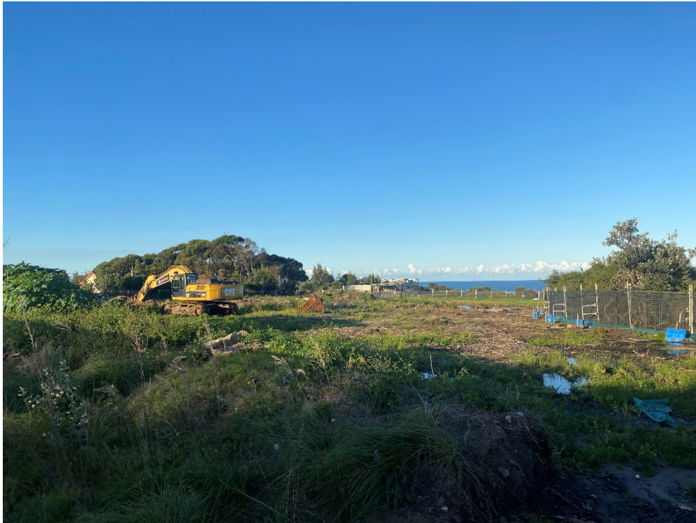
Figure 3 View of the cleared northern part of the site
